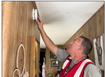
Rick Applegate installs a smoke alarm in a Meridian home. Teams installed 284 free alarms.
